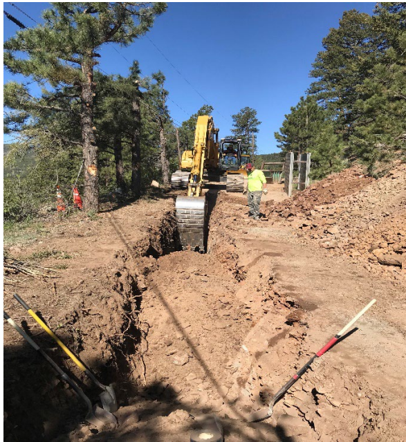
Timber Trail Road Main Replacement – construction crew at work
